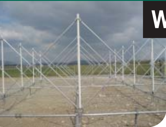
An array of 20 T3D quad antennas. Each antenna is around 1.3m wide and 2m high.
